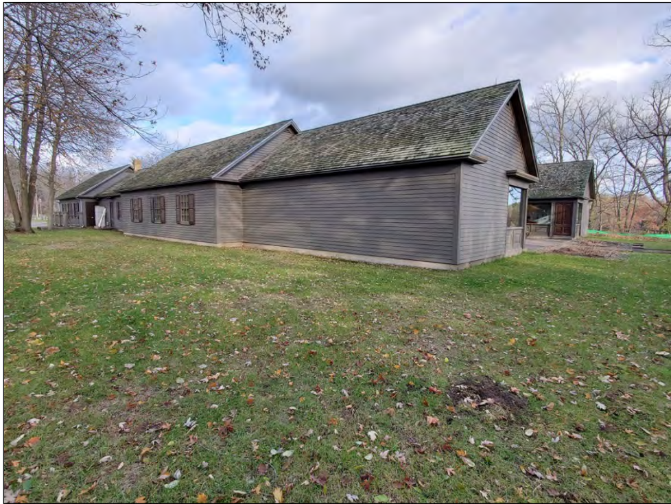
FIGURE 12. WEYERHAEUSER MUSEUM, WEST ELEVATION, 2023, LOOKING NORTHEAST
