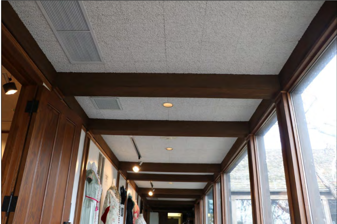
FIGURE 27. DETAIL OF CEILING, WEST EXHIBIT HALL, 2023
