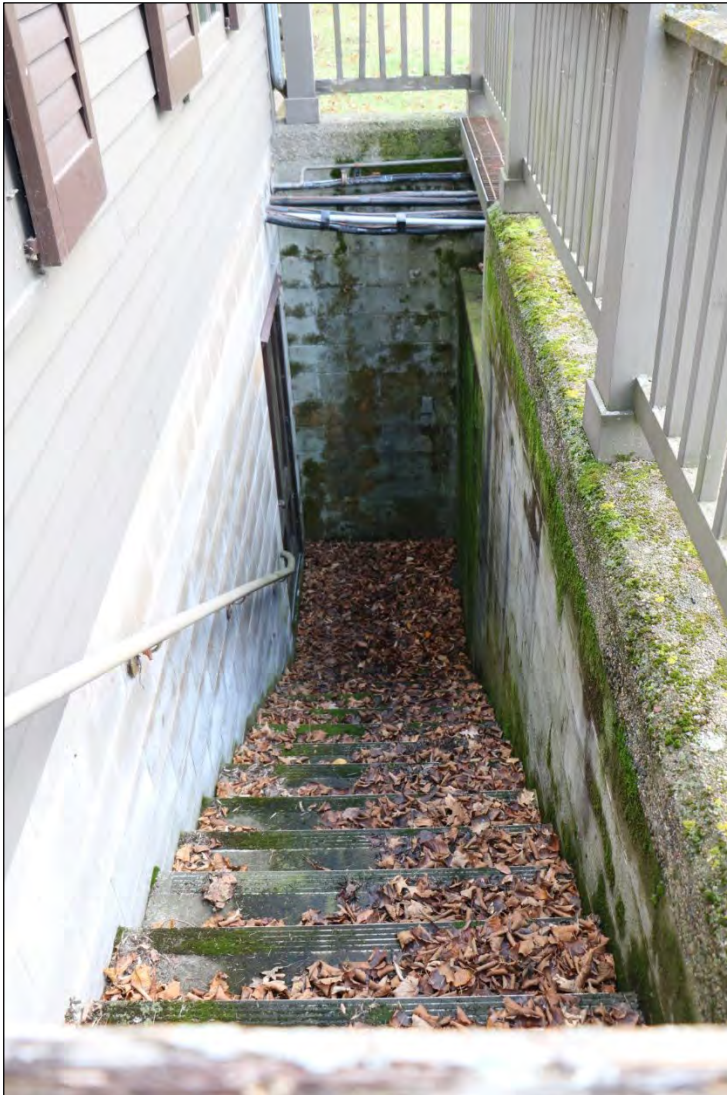
FIGURE 13. STAIRWELL AT BASE OF WEST ELEVATION OF SECTION E, 2023, LOOKING SOUTH
