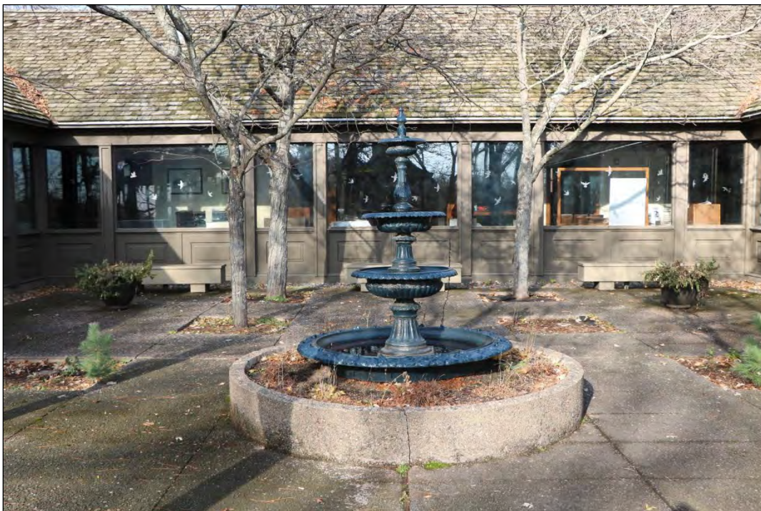
FIGURE 16. DETAIL OF COURTYARD-FACING ELEVATION, COURTYARD SURFACING, AND FOUNTAIN, 2023, LOOKING NORTH
