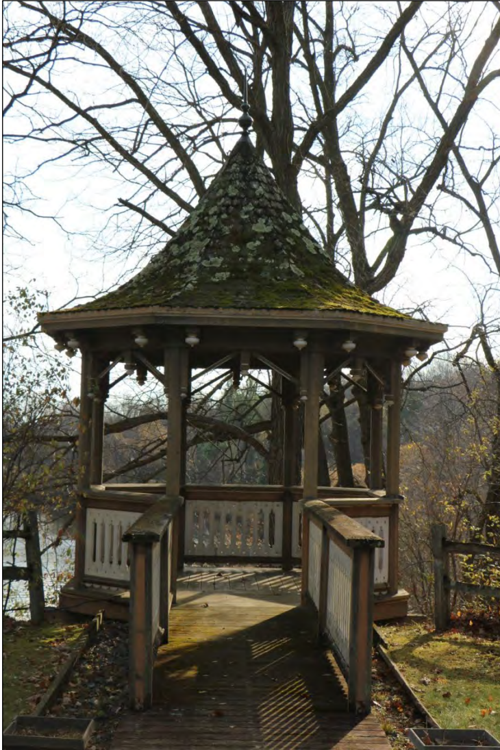
FIGURE 19. GAZEBO, 2023, LOOKING SOUTH
