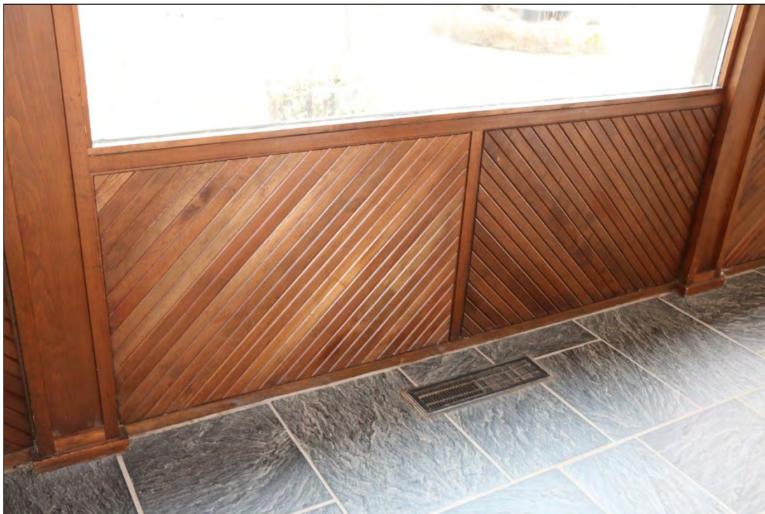
FIGURE 24. DETAIL OF BULKHEAD IN WEST EXHIBIT HALL, 2023, LOOKING EAST
