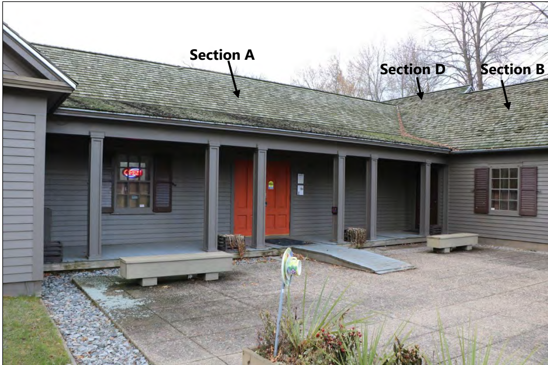
FIGURE 11. DETAIL AT FRONT ENTRANCE, 2023, LOOKING SOUTHWEST
