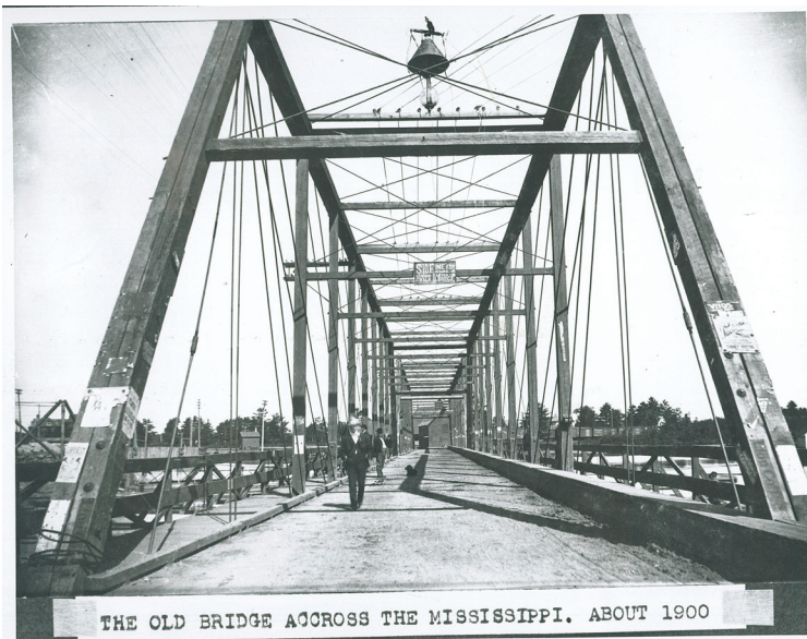
Wrought iron combination truss bridge across the Mississippi River at Little Falls, MN, built by Keepers & Riddell of the Milwaukee Bridge and Iron Works Company in 1883/1884. Photo c. 1900.
